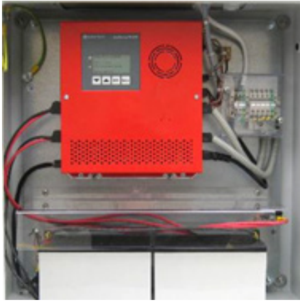
TK 250-500-750 with 2 batteries
