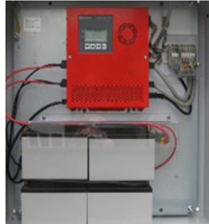
TK 1000 with 4 batteries
